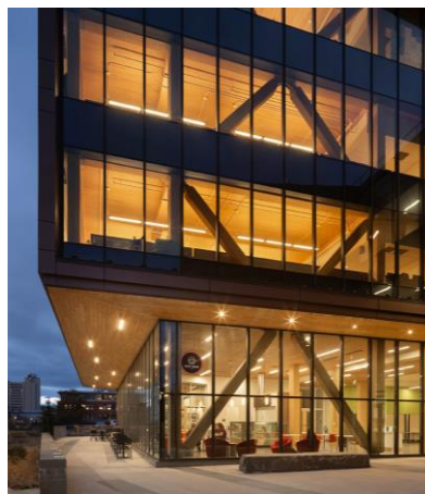
Figure 1. A chevron-type BTF: during construction (left) and in a finished building at night (right). (Photos courtesy of Nordic Structures).
