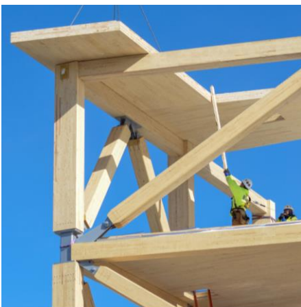
Figure 1. A chevron-type BTF: during construction (left) and in a finished building at night (right). (Photos courtesy of Nordic Structures).
