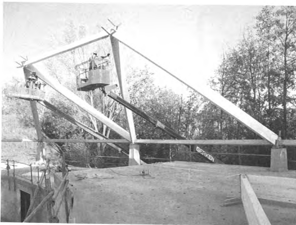
Fig 35 Two triangles of two beams, connected at the top. This is already a stable three-dimensional situation.
