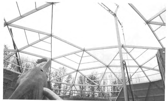
Fig 36 Each level of beams serves as a base for the next level
