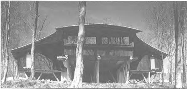
The buildings that result from these constraints are examples of an interesting architectural form that might be termed “high-tech-low-tech”, where highly developed technical solutions such as the epoxy connection are combined with a very low-tech material, the thinning, that is left almost entirely unprocessed to produce a novel form of building that simultaneously evokes the aesthetic of flying saucer and the nomadic hut.
