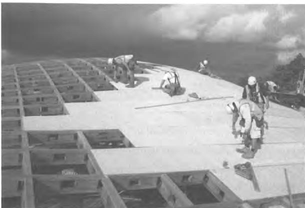
To act as a shell, the structure must be strong and stiff in its plane. Initially the concept included steel cables to triangulate and thus brace the shell in its plane. To save cost and make a more elegant structure the cables were omitted and the plywood covering, which is needed to support the raised seam roof, was used instead. In supporting roof loads, this in-plane structure is just as important as the more visibly obvious laths.
