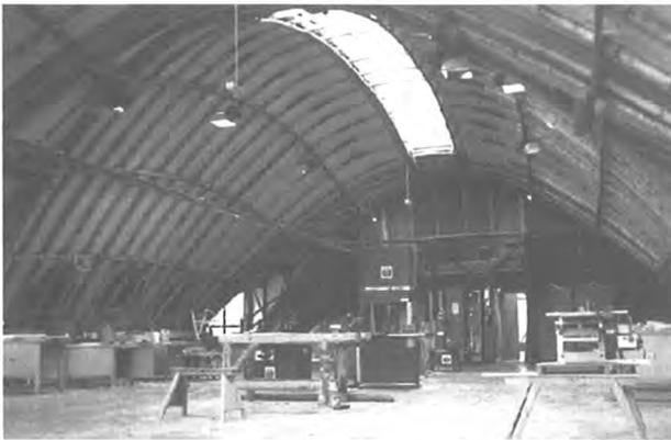
a curved arch. A splice piece was required at the crown to complete a smooth curve. The building was covered with a pre-patterned double layer membrane which provided additional bracing to the arches.
