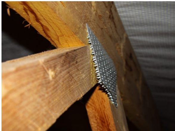
Figure 1.1. PMPF detached from the timber member
