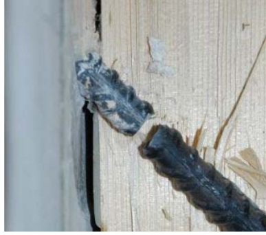
Fig. 6: Fatigue failure mechanism -X-connector
