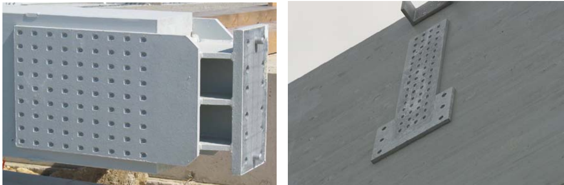
Figure 1: Examples of joints with inclined screws and steel plates as outer members
