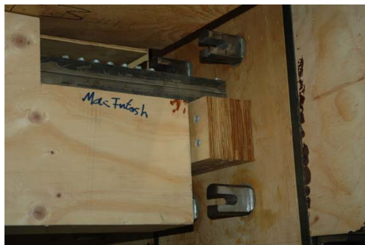
Figure 2. Hanging Beam/Floor Joist Connections
