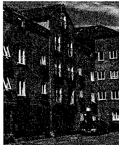
Figure 2 Five Storey Timber-Framed Apartments in South Wales
