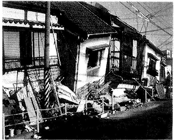
Photo.2 - Houses whose first story collapsed.
