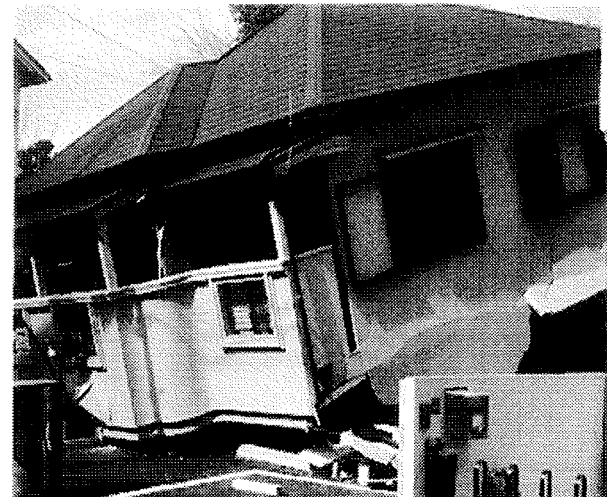
Photo.4- Collapse of newly constructed house. The first story was garage and the displacement of shear wall was eccentric.
