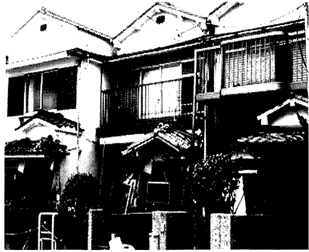
Photo.8 - Damage of the first story. No shear walls were placed in front of the house.
