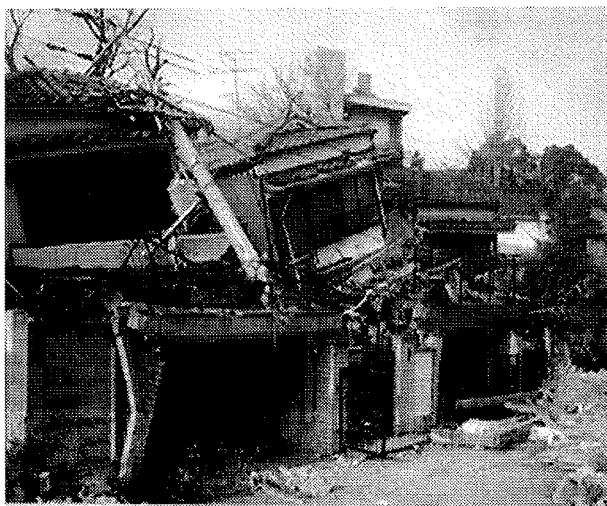
Photo.6 - Collapse of the second story. The first story was a garage of reinforced concrete.
