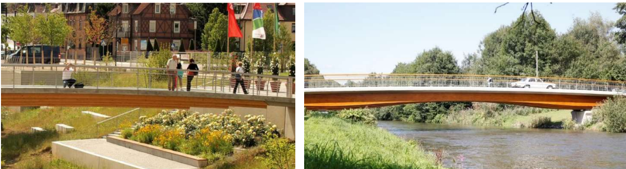
Figure 1.2. TCC-bridge with 27.7 m span in Schwäbisch Gmünd, Germany build in 2012 (left) and TCC-bridge with 28 m span in Lohmar, Germany build in 2014 (right), sources: IB Miebach and M. Gerold
