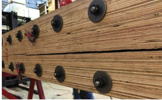
Figure 16. MPP casing split resulting from strong axis steel core buckling.
