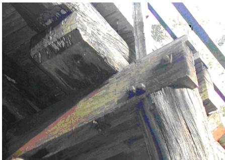
Figure 4: Load transfer by perpendicular to grain stresses
