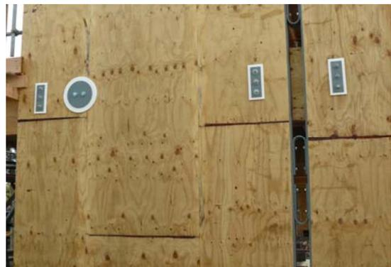
**Figure 7.** Shear walls showing the cylindrical shear connector with Teflon spacer, slotted location bolts, and U shaped yielding steel energy dissipaters
